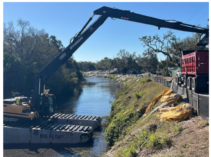
Stormwater clears 100,000 cubic yards of sediment from Phillippi Creek.
