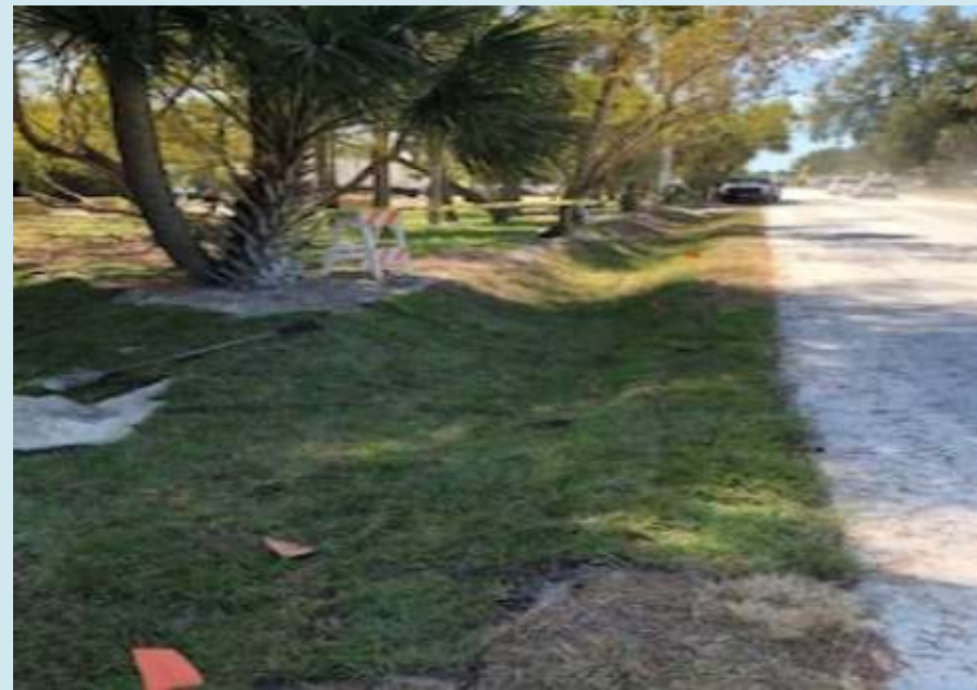
New drainage ditch along Casey Key Road.
