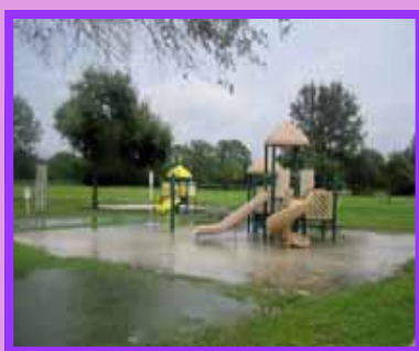
Flooding in the play area
