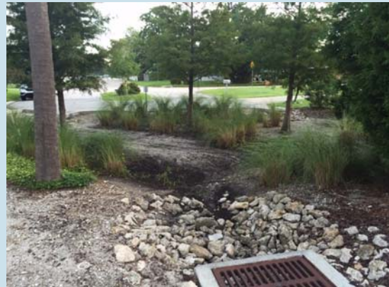
Gold Avenue bio swale planting.
