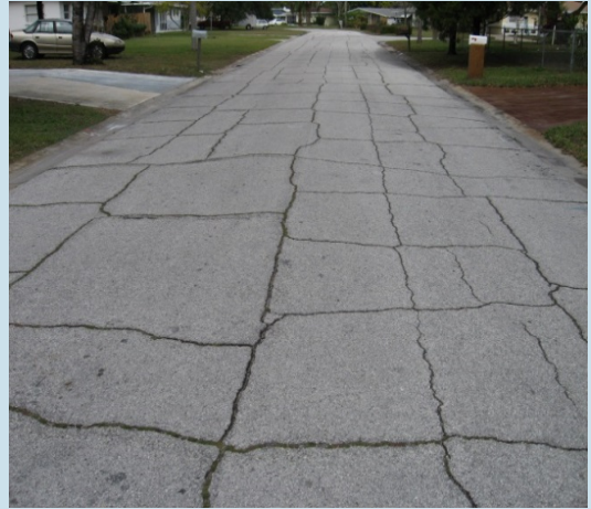
Kensington Park roadway before resurfacing project.
