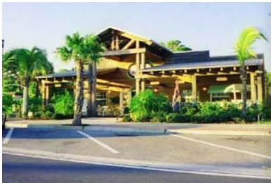
Existing commercial structure on Dearborn St.
