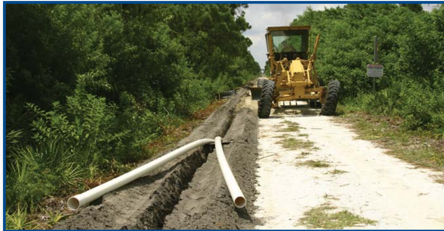
Gibbs & Register placing two 4" telecommunication conduit.
