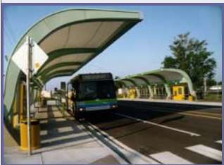
Miami-Dade Busway Station
