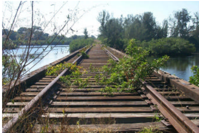
Railroad Trestle Over Curry Creek
