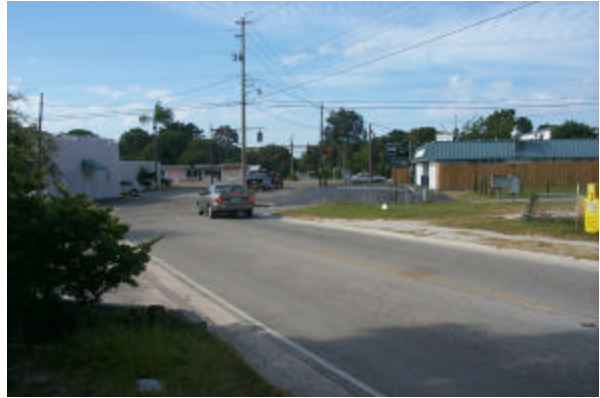
Colonia Lane will be reconstructed in FY 2005
