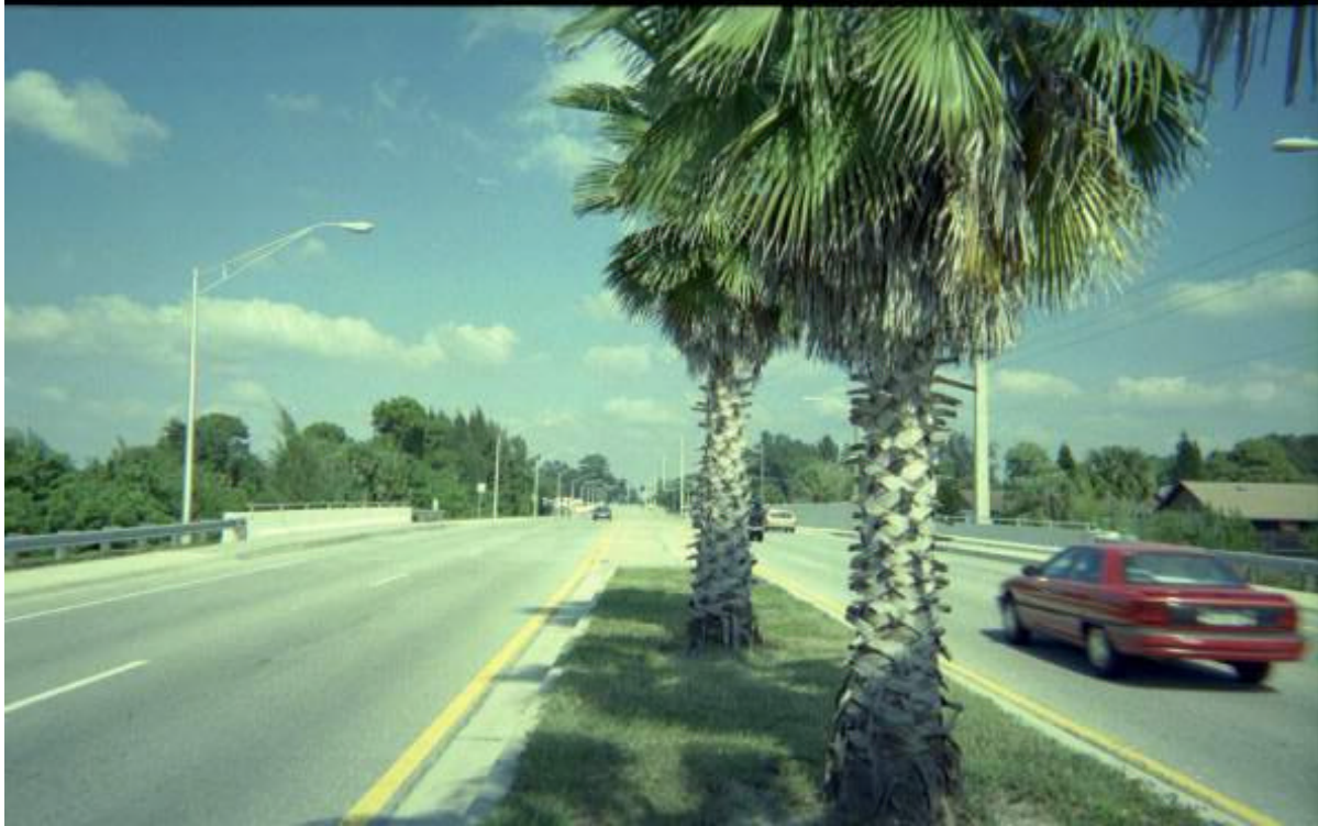
Albee Farm Road is an Arterial Roadway with Sidewalks, Bike Lanes, Medians and Landscaping
