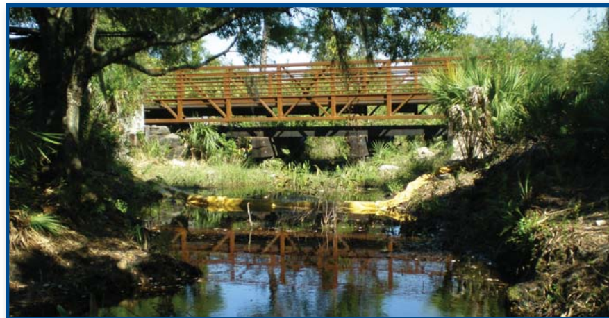
History meeting future with the placement of the first prefabricated bridge.
