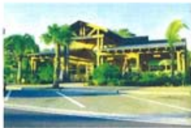
Existing commercial structure on Dearborn St.
