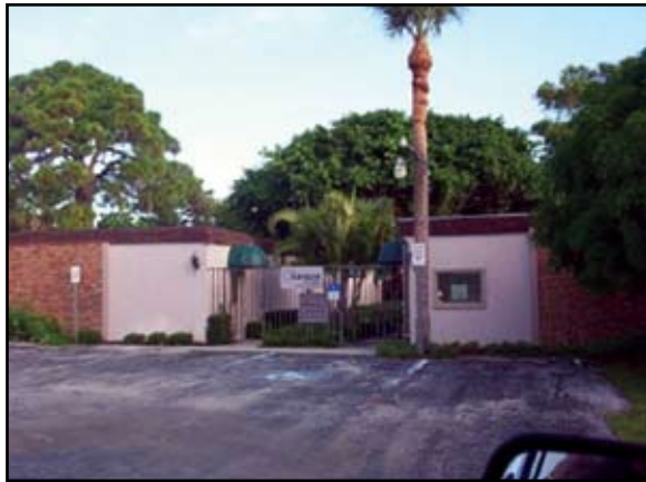
Banyan Court Before
