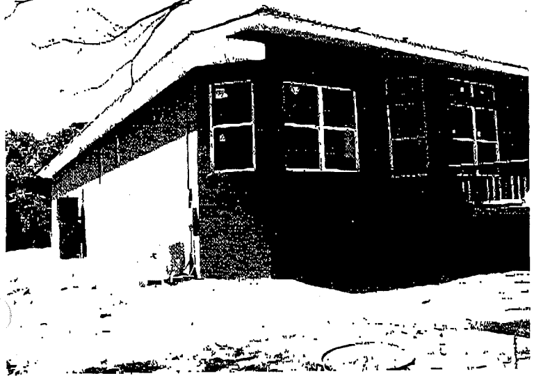
FIGURE 3 - REAR / RIGHT SIDE VIEW
