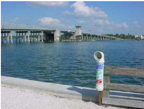
North Siesta Key Bridge
